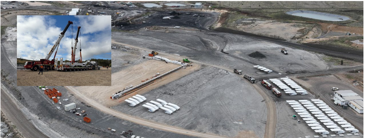
Longwall machinery "Mini-build" at the Maxwell mine
