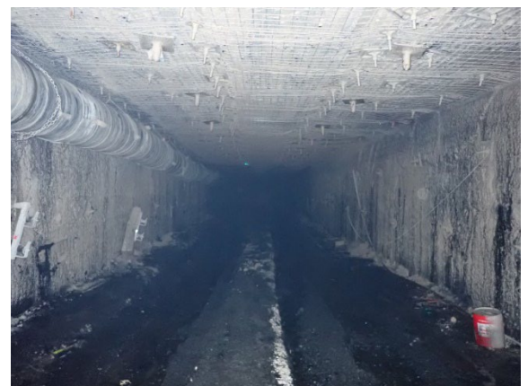
A “development road” driven at the Longwall Operation
