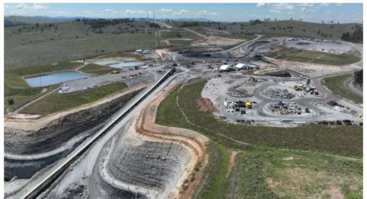
Underground mine entry area (MEA). Note progressive establishment of vegetation and pastures within the MEA
