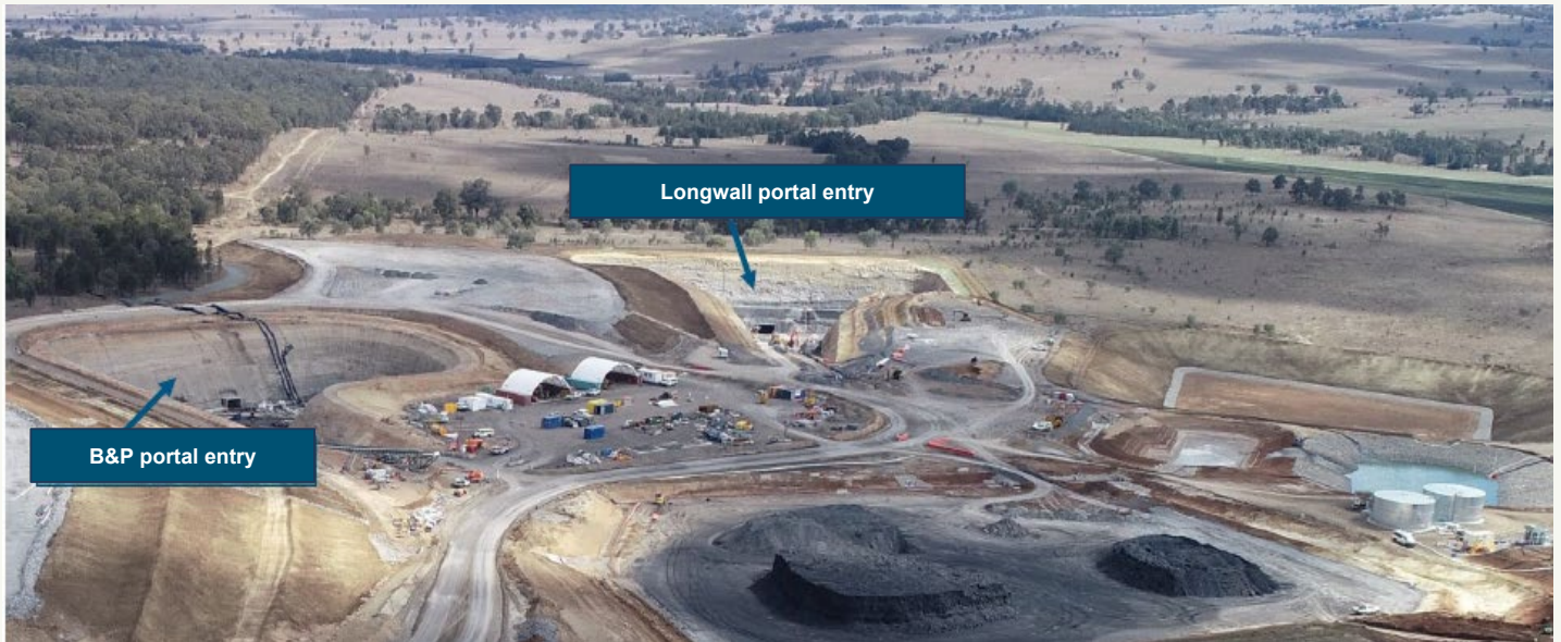
Photo: Mine Entry Area (MEA)
