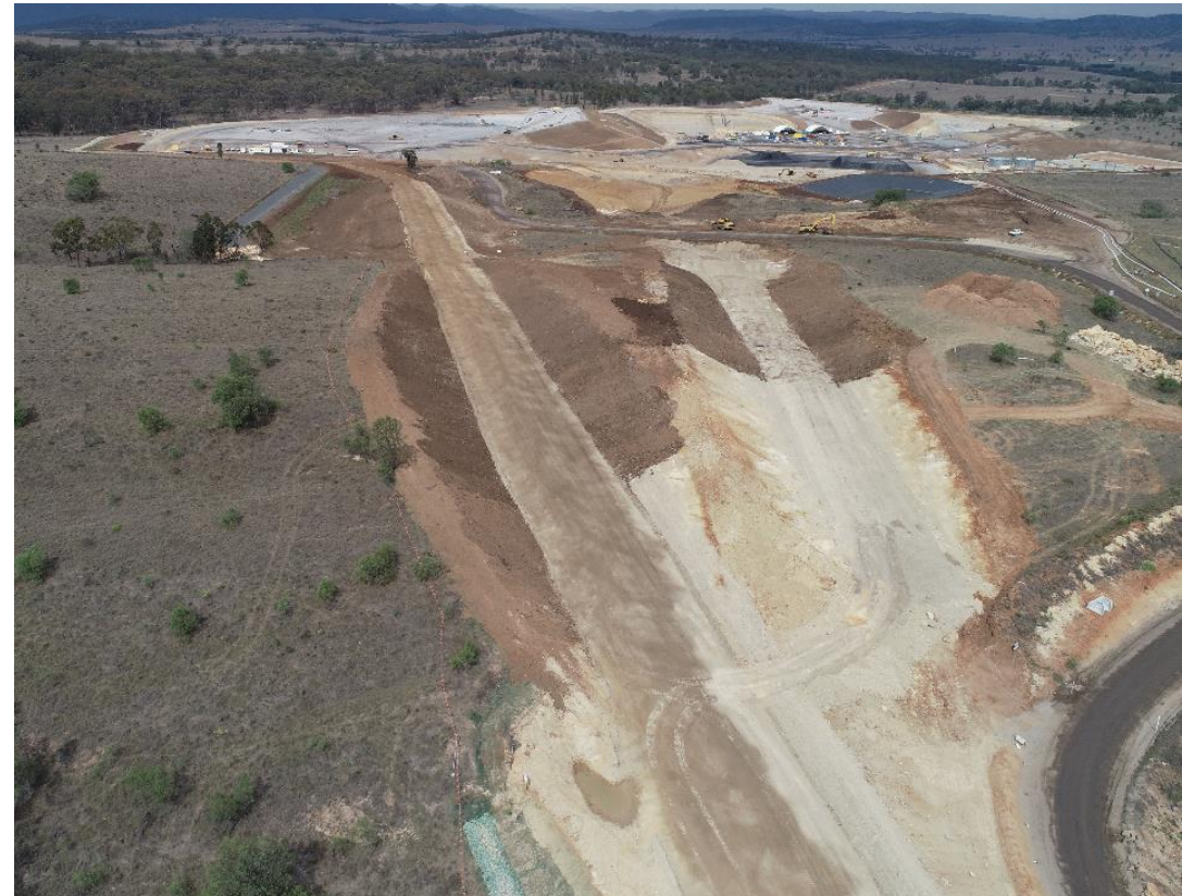
Conveyor Trace – October 23
