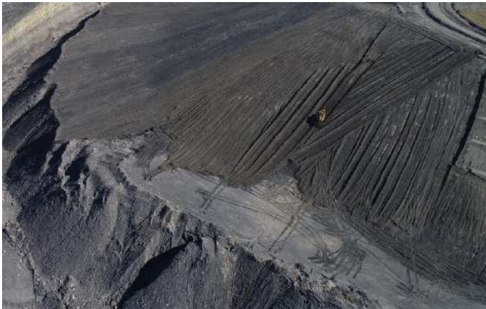
Reshaping with Dozer
