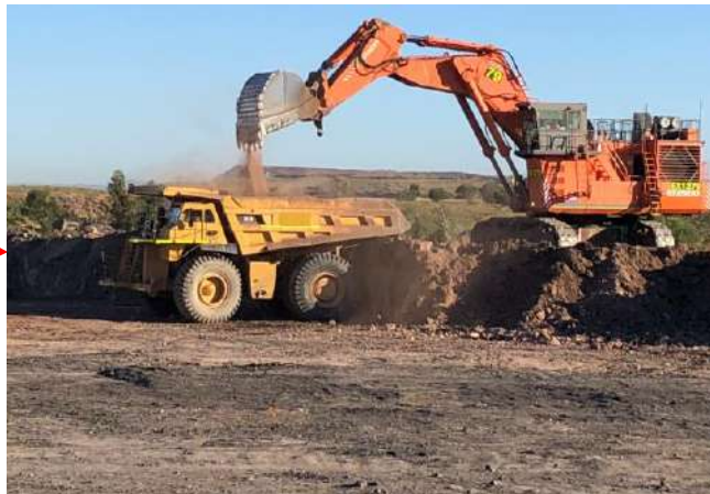
Haul and spread inerts
