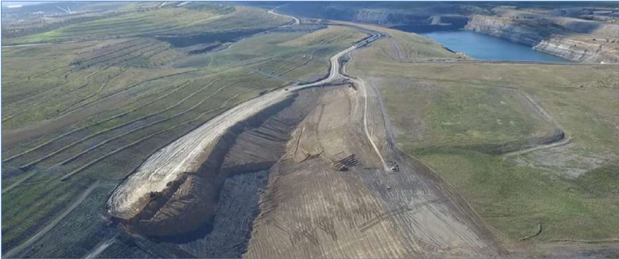
Plate 7 – Rehabilitated Maxwell Infrastructure Waste Emplacement – August 2019
