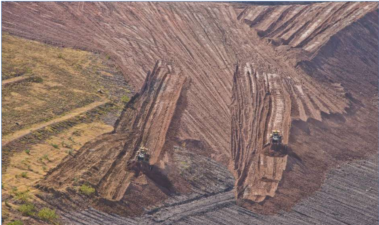
Plate 4 – Dozers Spreading Inert Capping Material for Rehabilitation
