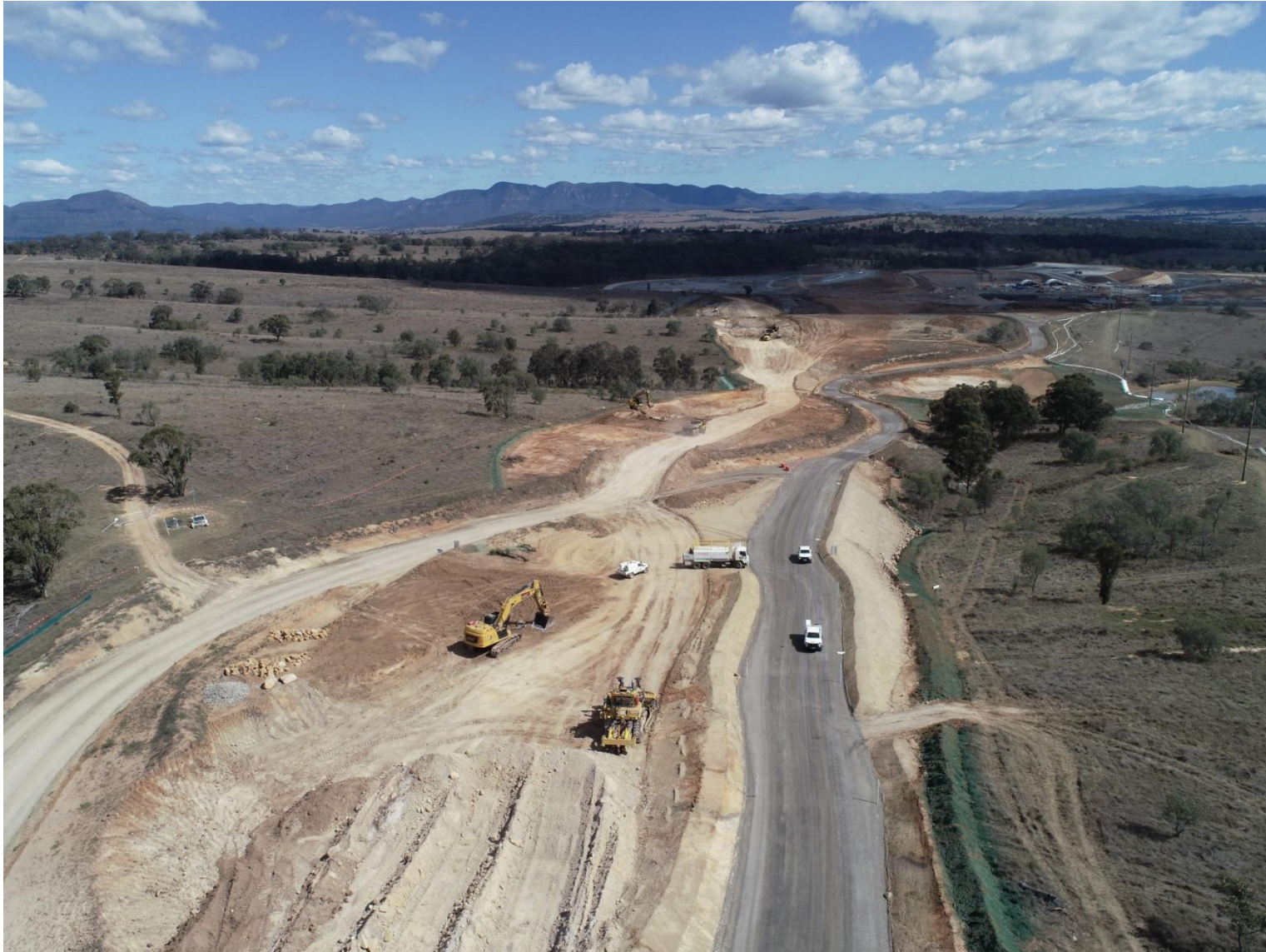
Access Rd Construction
