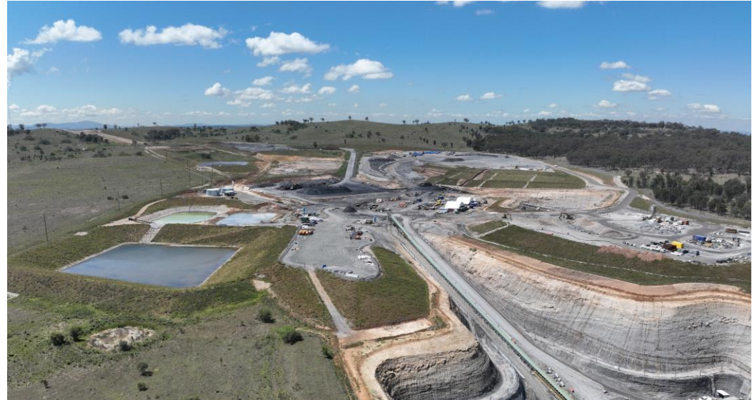
Underground entry area Oct 2024
