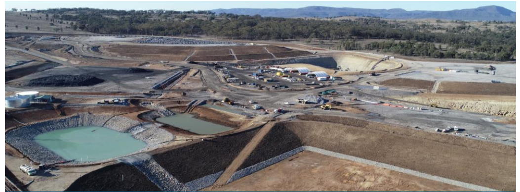
Underground entry area last year
