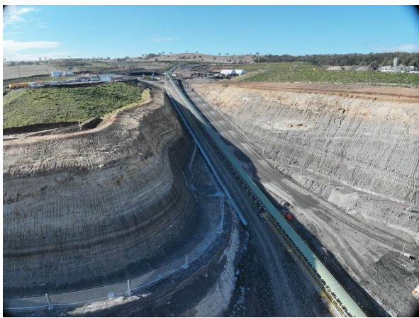
Longwall drift conveyor
