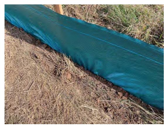
Plate 36 - Sediment fence installed to temporary access track prior to permanent road construction
