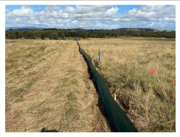
Plate 35 - Sediment fence installed to temporary access track prior to permanent road construction
