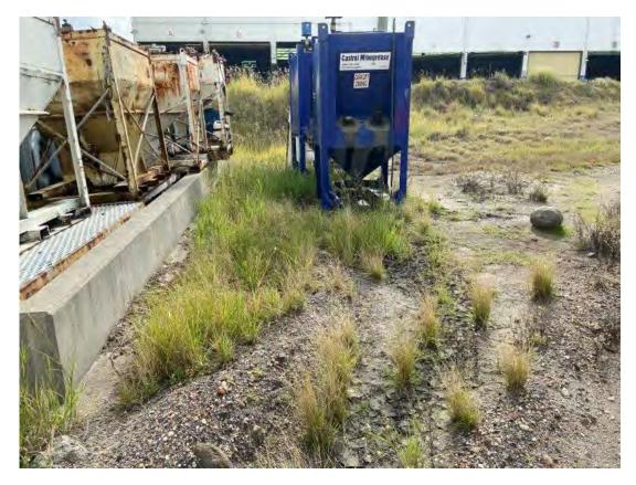
Plate 24 - Leaking fuel pod outside of bunded area
