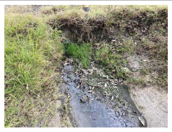
Plate 19 – Under road pipe blocked leading from wash bay to oily water separator
