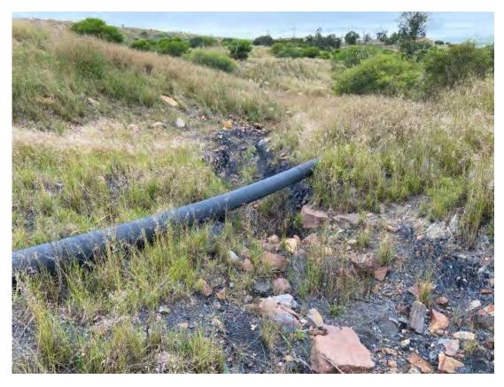
Plate 48 - Evidence of gully erosion through dirty water drainage channel to southern void
