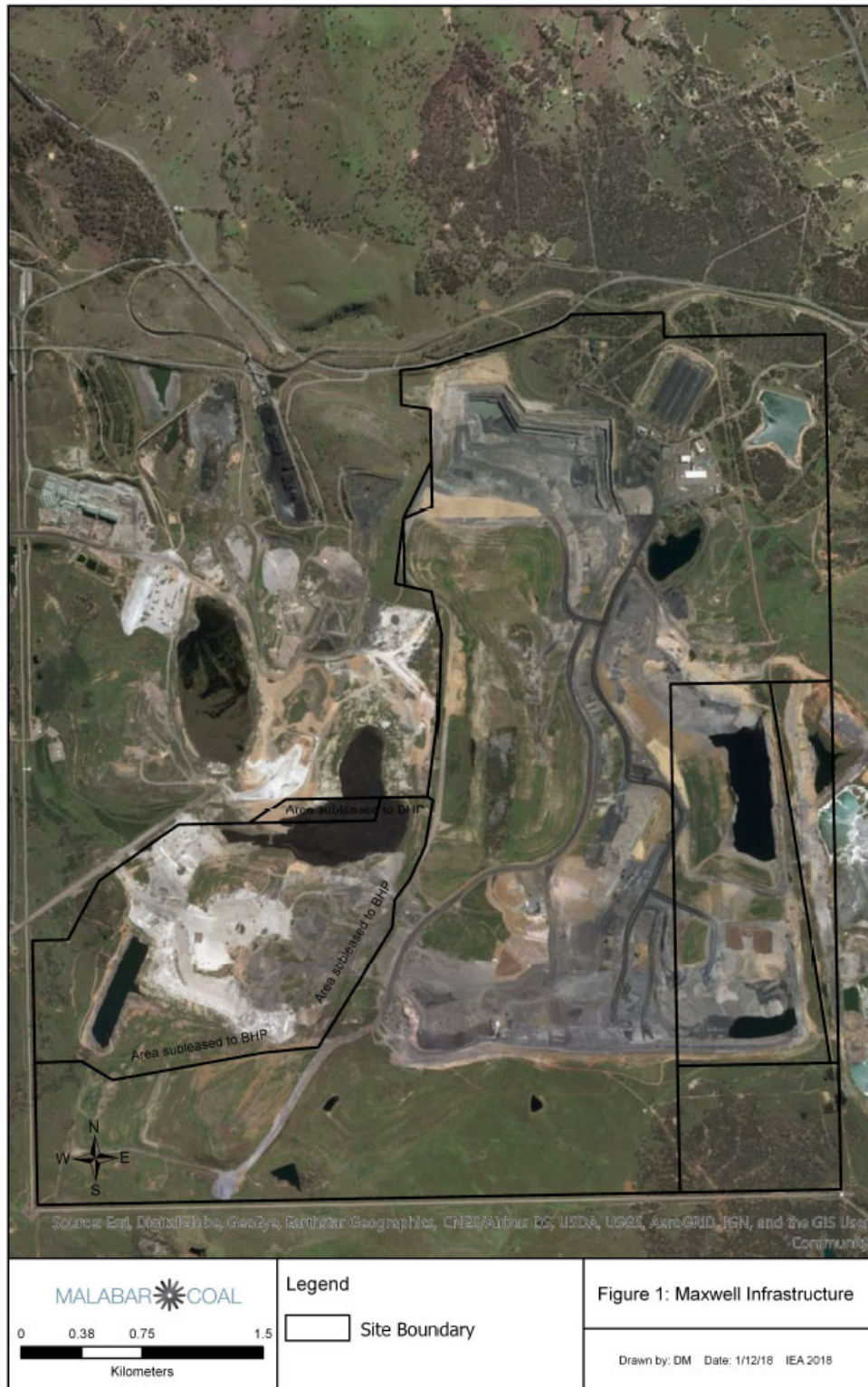
Figure 1 Maxwell Infrastructure Site
