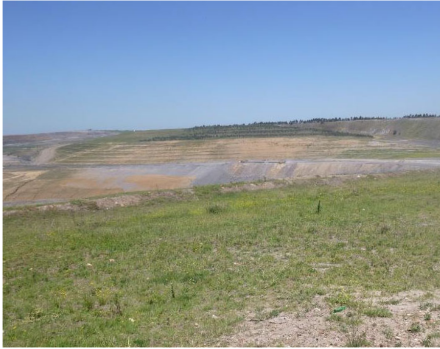
Photo 5 – Some contour drains have not been designed and constructed as per the Water Management Plan commitments
