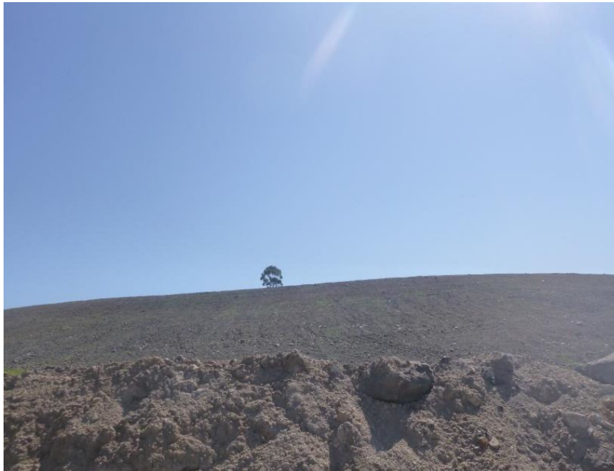
Photo 8 – Newly rehabilitated area has not been deep ripped on a horizontal contour. Chisel plow has been used instead. This may lead to increased erosion in the future.
