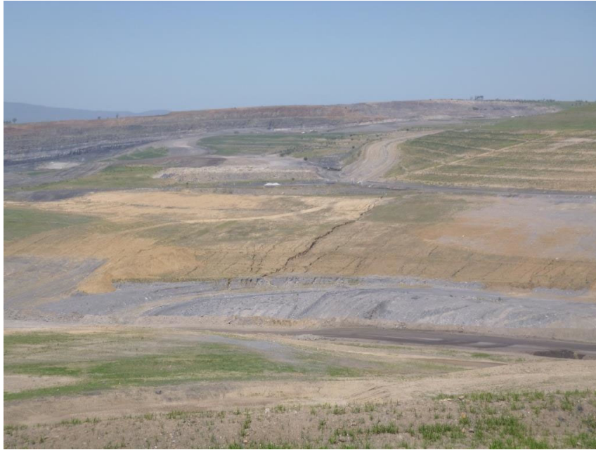
Photo 7 – Large area of gully erosion. It is proposed that a drop structure will be designed and constructed in this section of rehabilitation.
