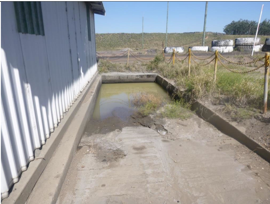
Photo 22 –Sediment to be removed from the lube bay and moved to the landfarm area
