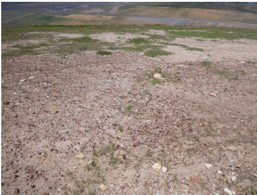
Photo 4 – Some areas of existing rehabilitation require remedial works
