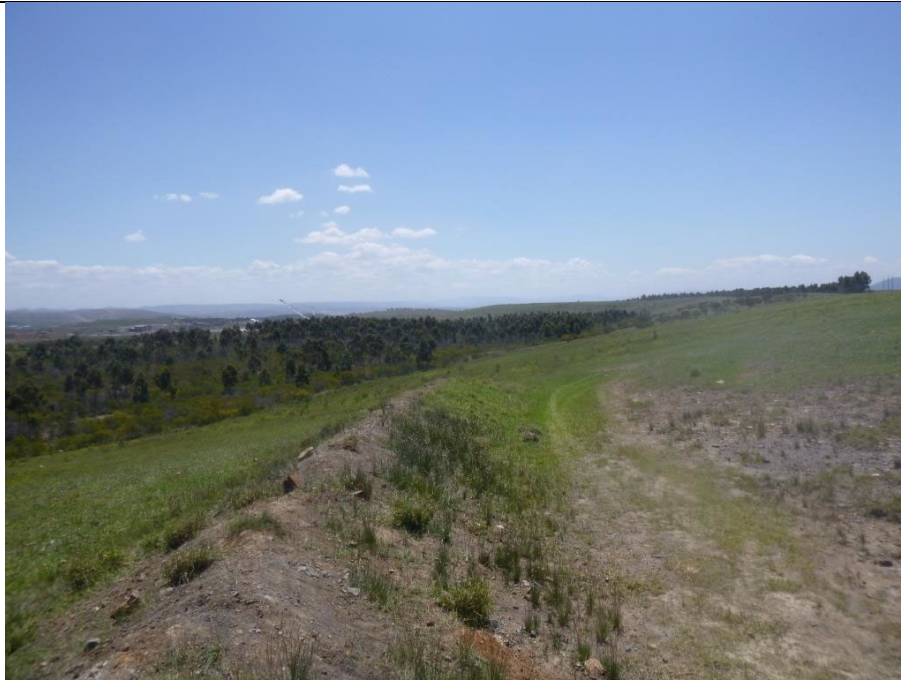
Photo 17 – Bund designed as per the Water Management Plan
