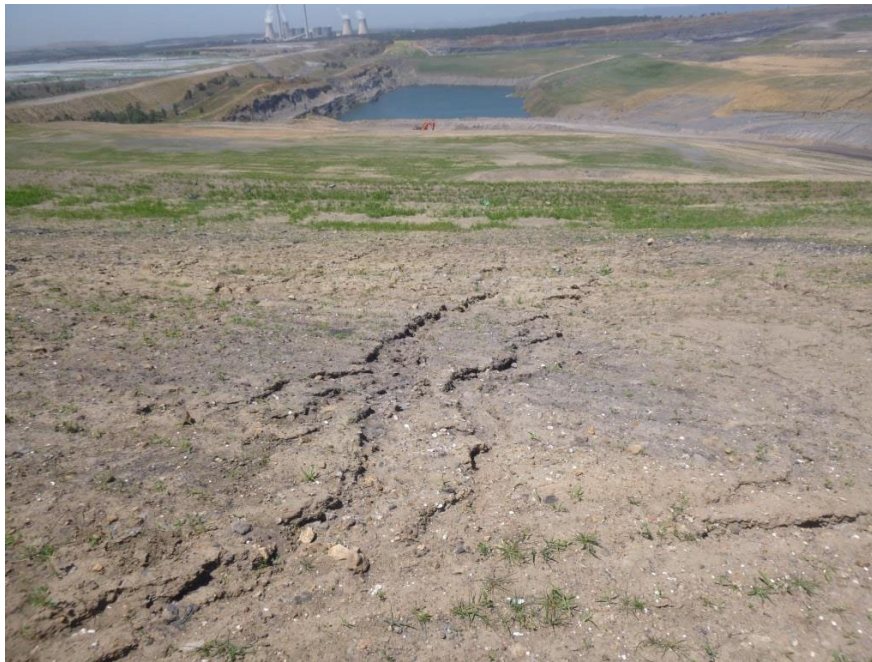
Photo 10 – Areas of erosion in sections of rehabilitation which have not been deep ripped.
