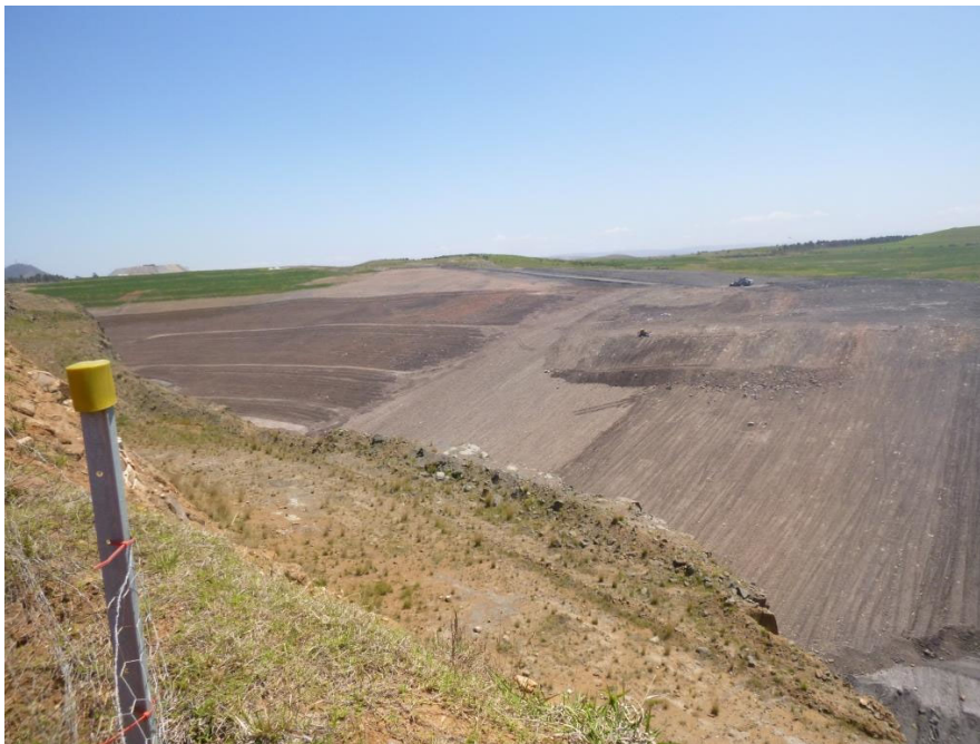
Photo 12 – Areas of rehabilitation currently being shaped
