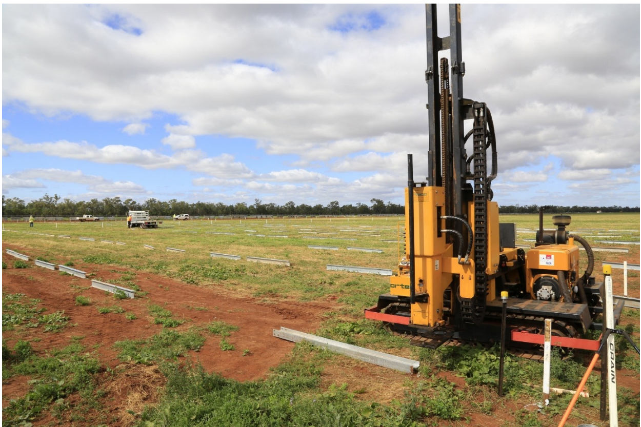
Figure 4-4 Typical pile driving unit (Image courtesy of PARF)
