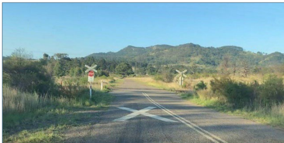
Plate 6-1 – Level Crossing on Antiene Railway Station Road
