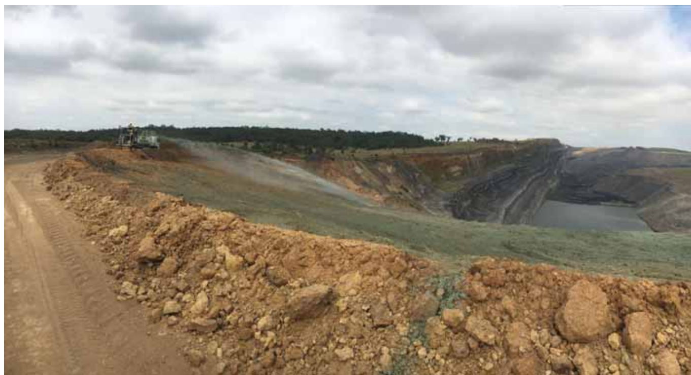
Plate 1 Hydro-mulching SPW Highwall
