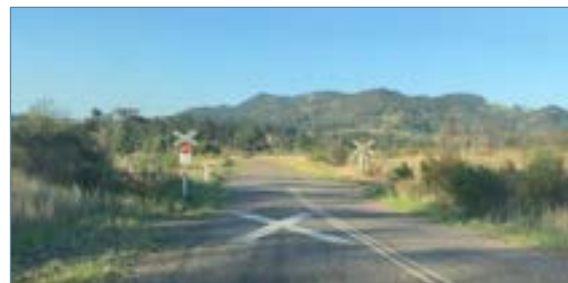
Plate 6-14 – Level Crossing on Antiene Railway Station Road
