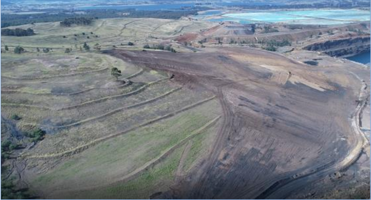
Plate 2 – Rehabilitated Maxwell Infrastructure Waste Emplacement – September 2018
