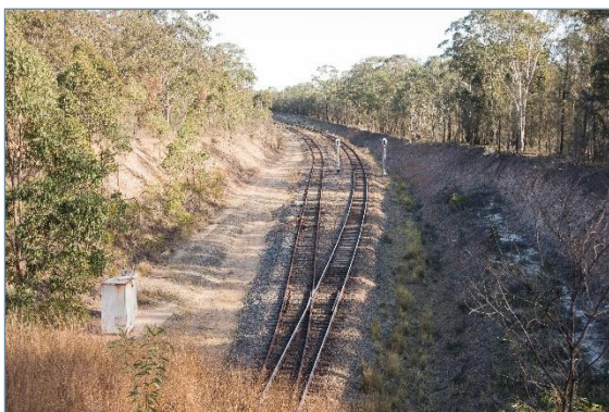
Plate 2-4 – Antiene Rail Spur
