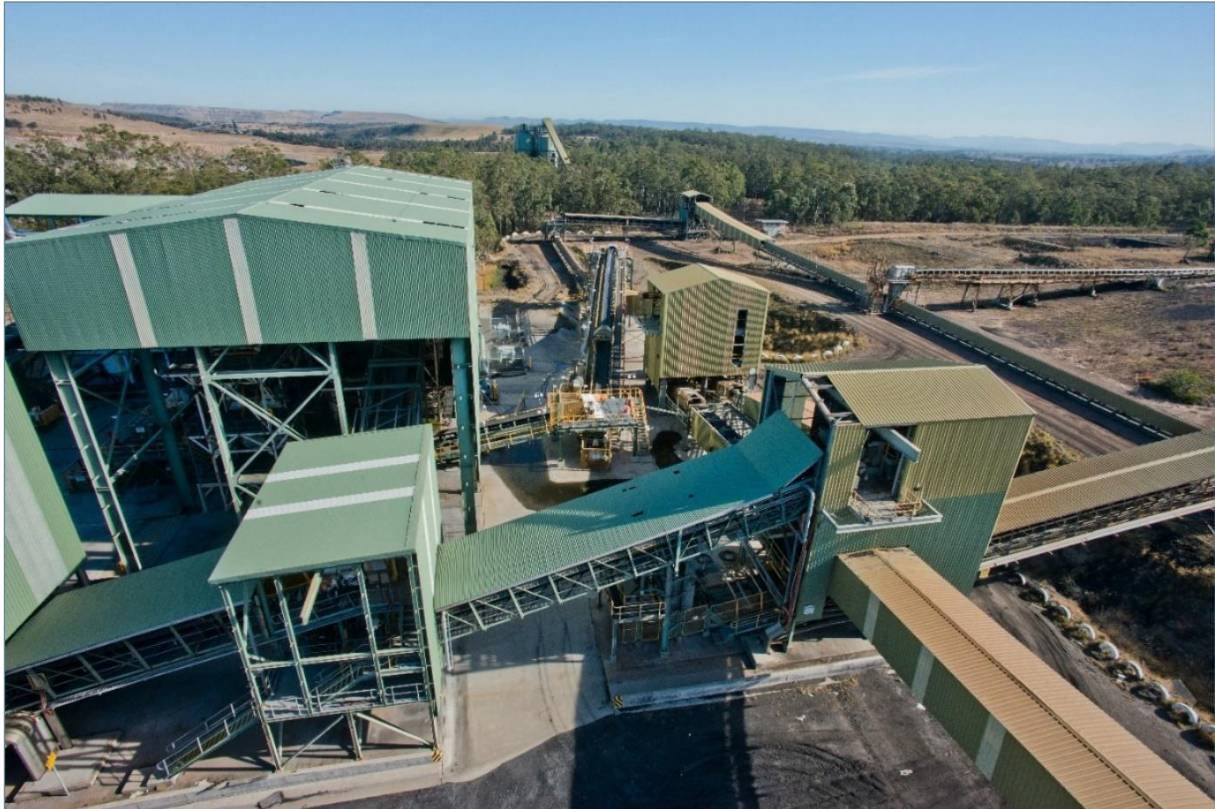
Plate 2-2 – Existing Maxwell Infrastructure
