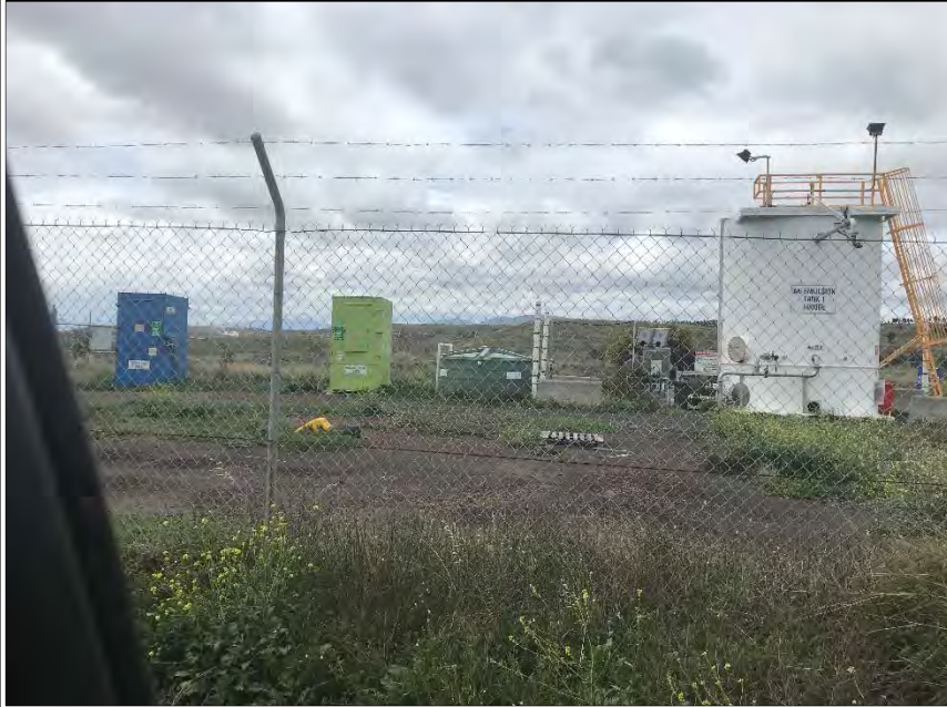
PHOTOGRAPH AL: MAXWELL INFRASTRUCTURE, AMMONIUM NITRATE EMULSION AST
