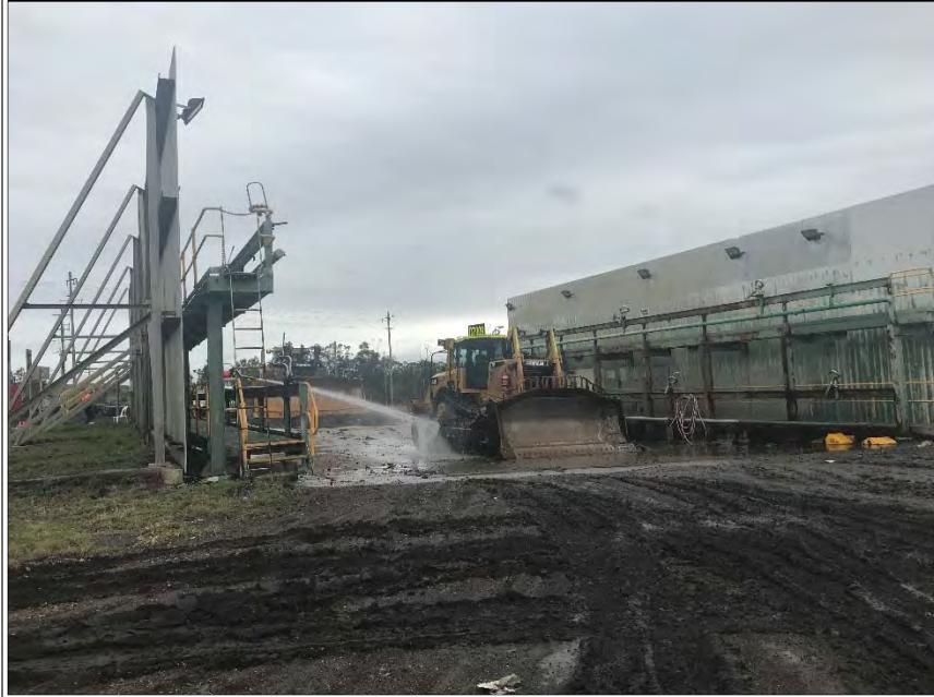
PHOTOGRAPH AH: MAXWELL INFRASTRUCTURE, HEAVY VEHICLE WASH DOWN BAY
