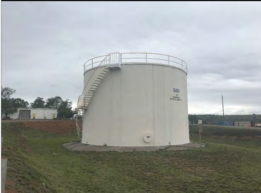
PHOTOGRAPH AI: MAXWELL INFRASTRUCTURE, 860 000 L DIESEL AST
