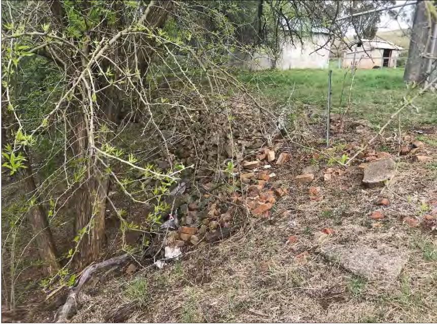
PHOTOGRAPH U: BUILDING AND DEMOLITION WASTE STABILISING CREEK BED
