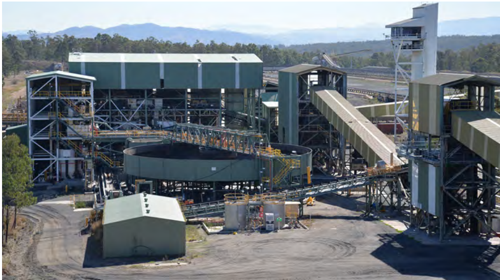
Existing CHPP, workshops and coal loading equipment at Maxwell Infrastructure facility.
