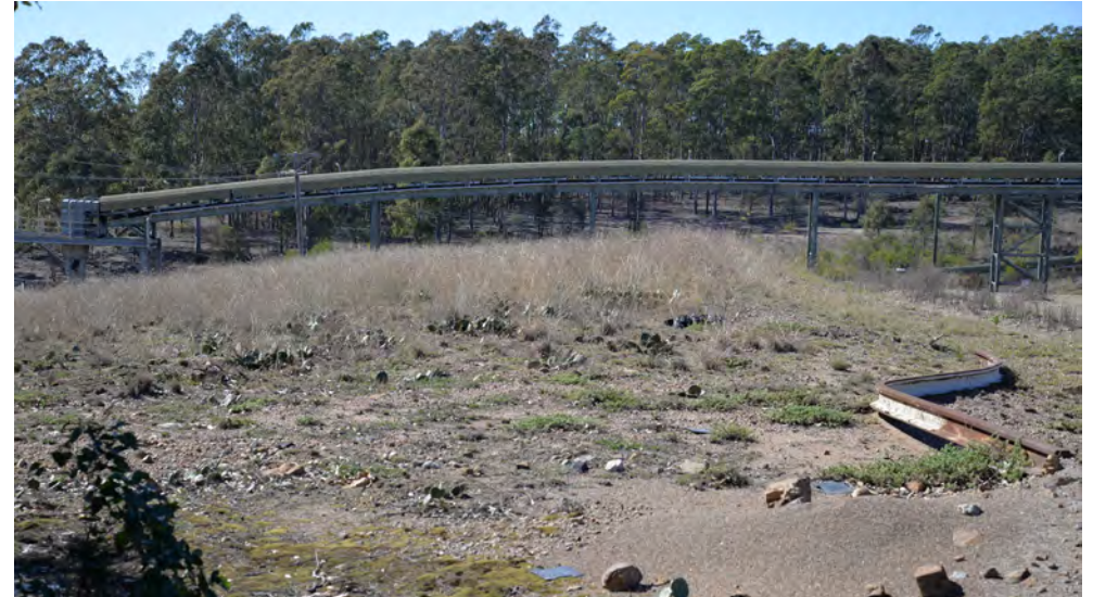
Existing overland conveyor at Maxwell Infrastructure facility uses muted colours borrowed from surrounding vegetation thereby reducing its contrast and visual effects.
