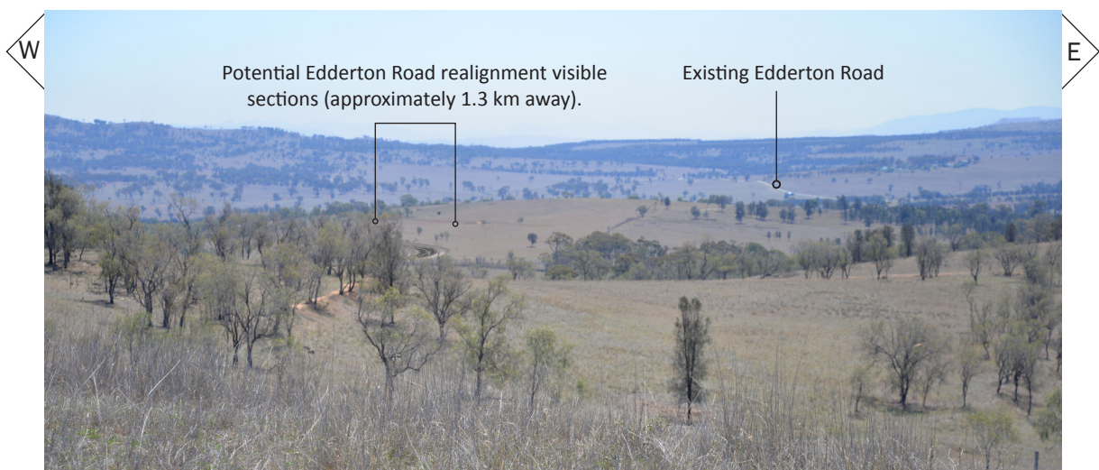
Existing view with new road alignment filtered by foreground vegetation. Ridge line in middle ground screens the rest of the realignment in foreground.
