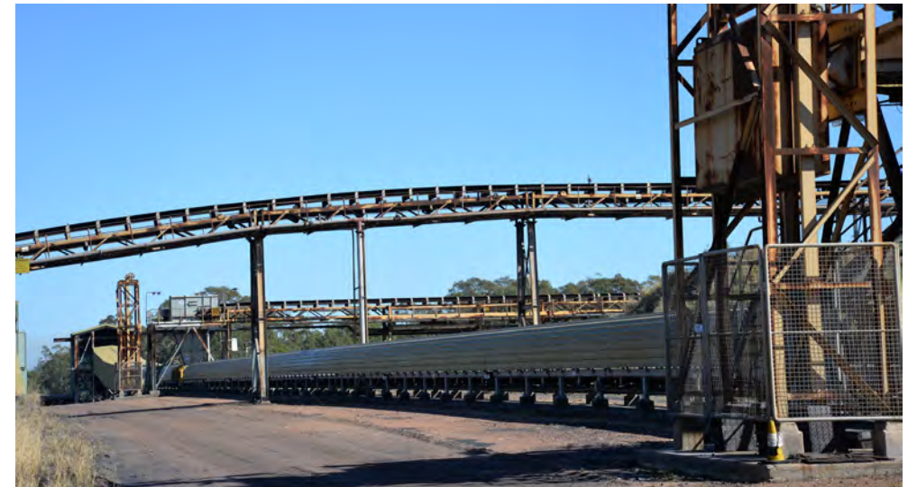
Existing coal processing and loading equipment.
