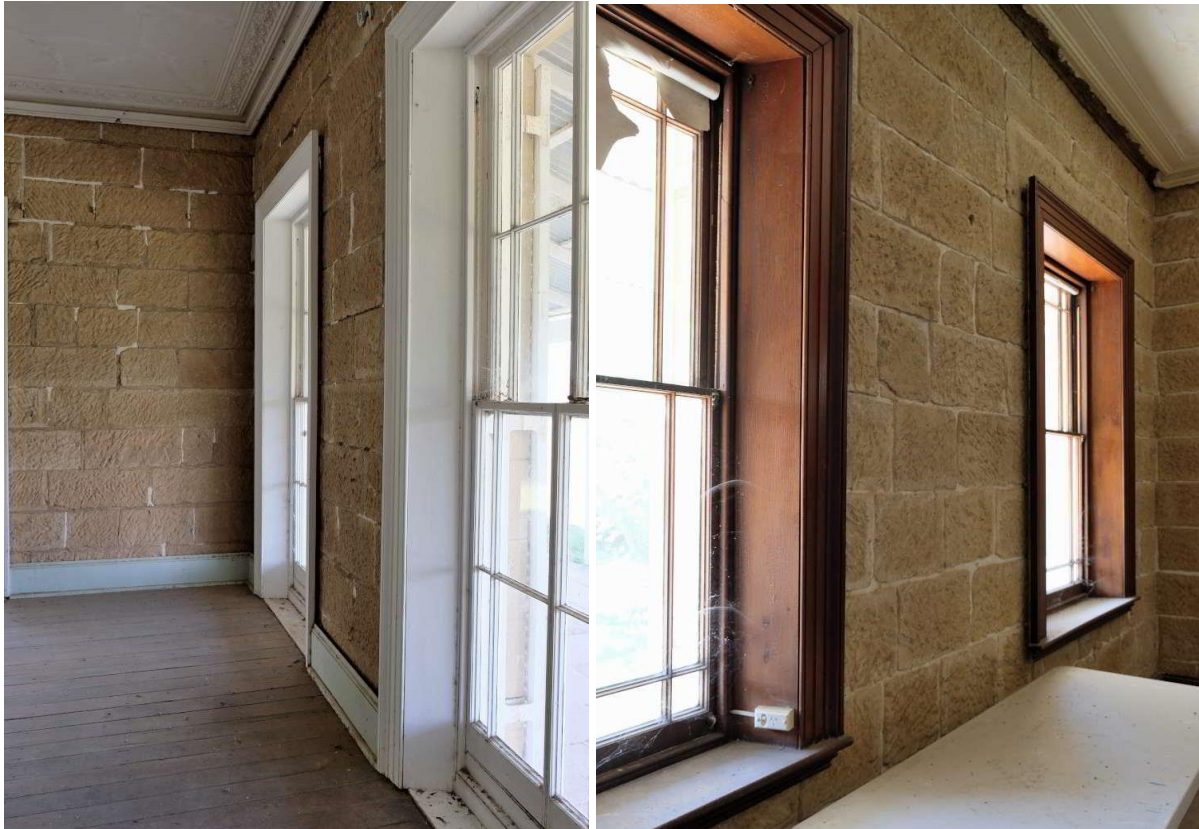
Figure 54 – Interior view of typical painted joinery (left) and clear finished joinery (right).
