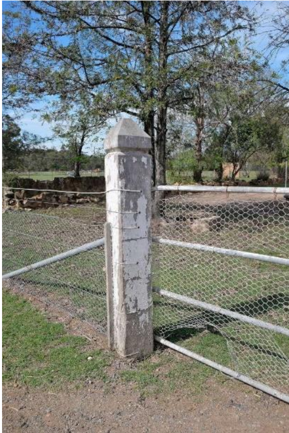
Figure 24 – Timber gate post at entry to yard of Bowfield Homestead.
