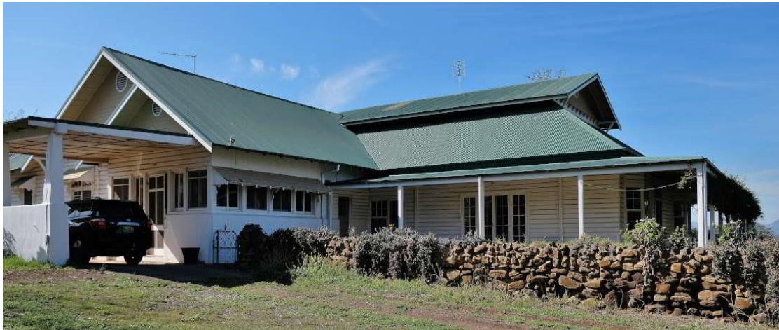
Figure 16 – South elevation with the ‘Porte Cochere’ at the left and original 1904 section to the right.
