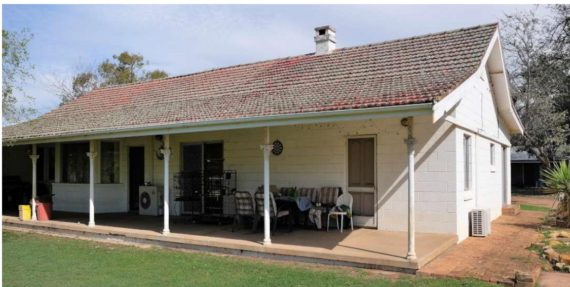
Figure 30 – View of the front wing of Bowfield Homestead, c.1960s.
