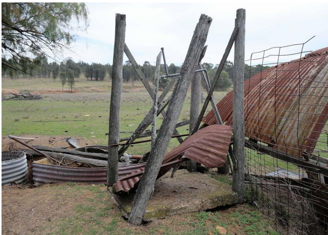
Figure 37 – Remains of four tall posts, two sides fitted with bracing, a concrete floor and galvanised water pipes, which are indicative of a shower shed having existed in this location.
