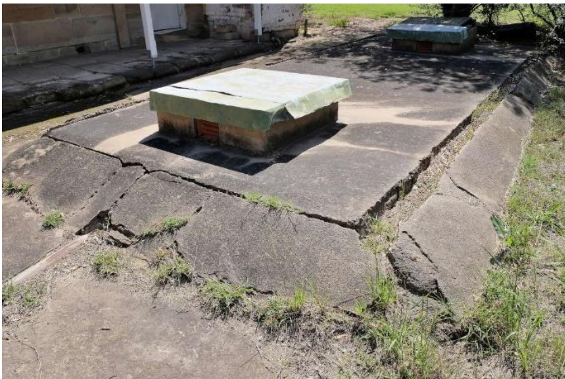
Figure 49 – The underground concrete-lined water tank located south of the rear wing.
