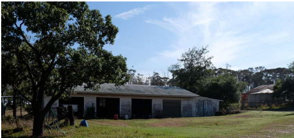
Figure 14 – View of the machinery shed at Edderton.
