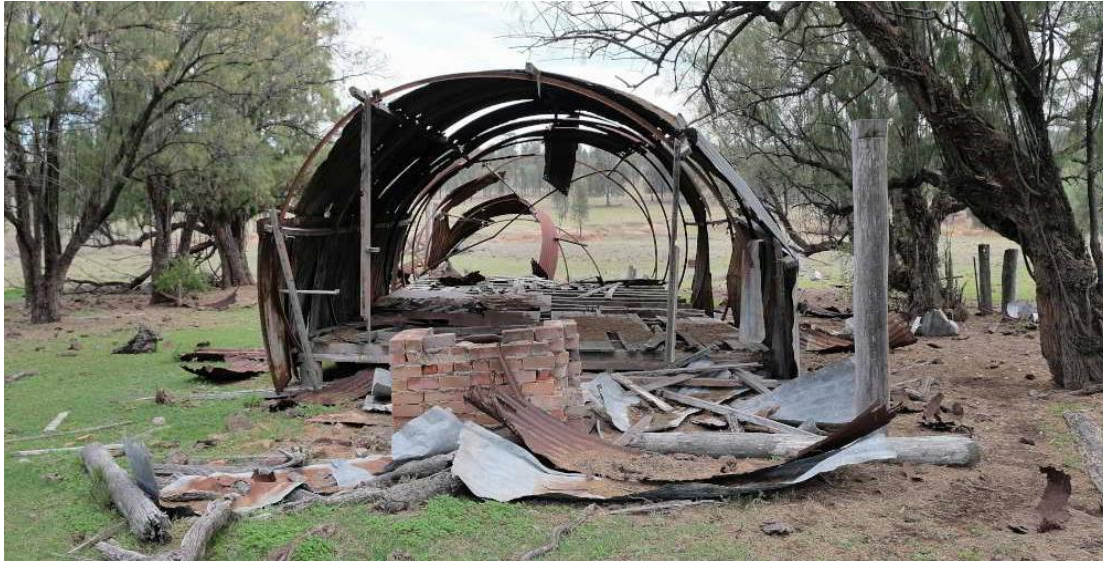
Figure 35 – View of the northern end of the Nissen Hut with the brick fireplace with plate for cooking.
