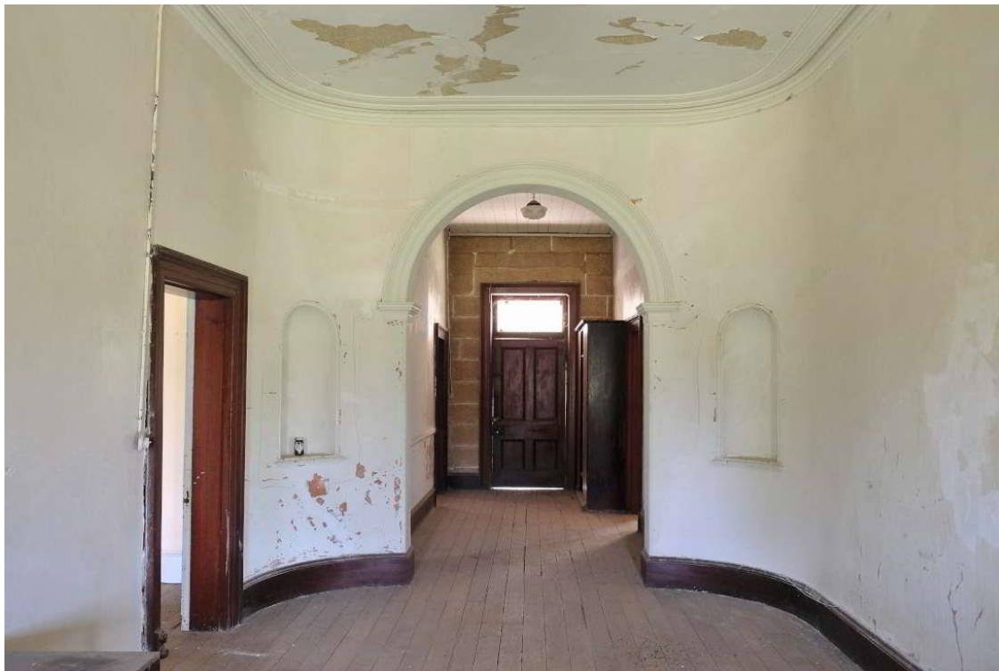
Figure 53 – Interior view of the rendered, curved walls and niches of the homestead's main entry.
