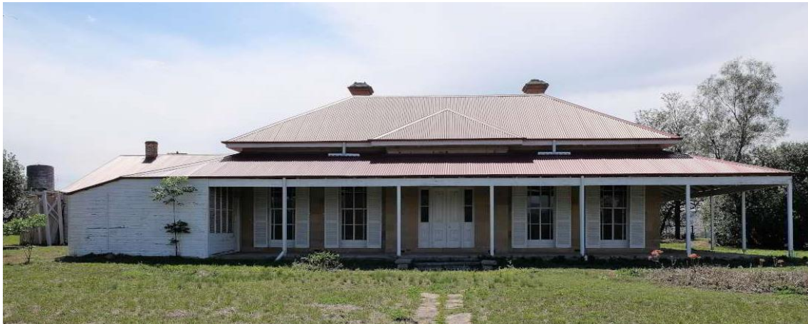
Figure 46 – View of the front of Plashett Homestead overlooking the Hunter River to the south-west.
