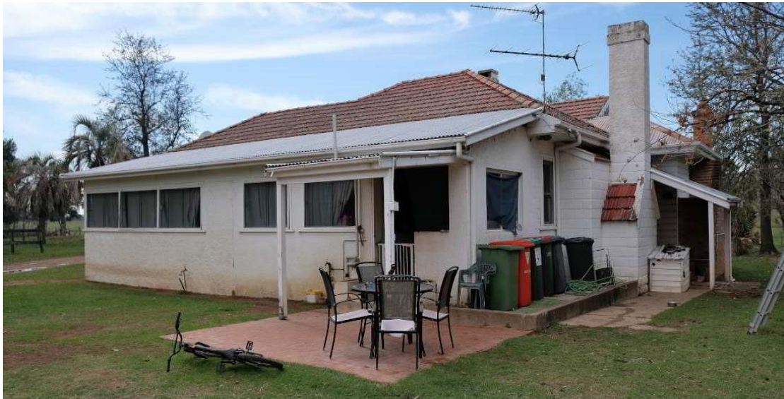
Figure 29 – View of the south-west corner of Bowfield, showing the hip roof of the second wing constructed in off form rendered concrete and chimney, as well as a more recent skillion roofed and enclosed addition of the homestead.
