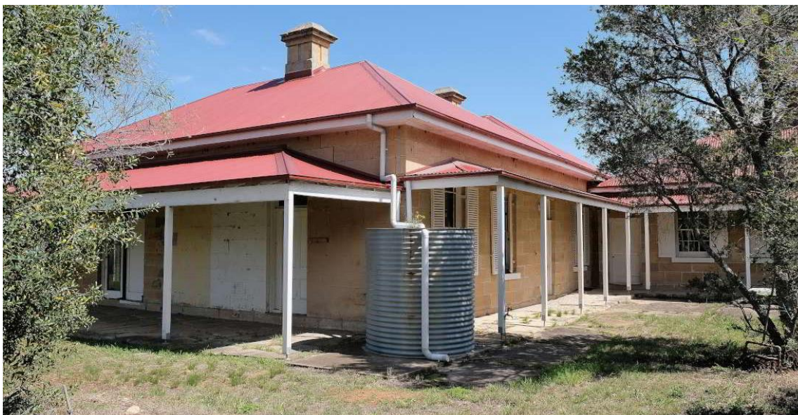
Figure 47 – View of the south-east corner of Plashett Homestead.
