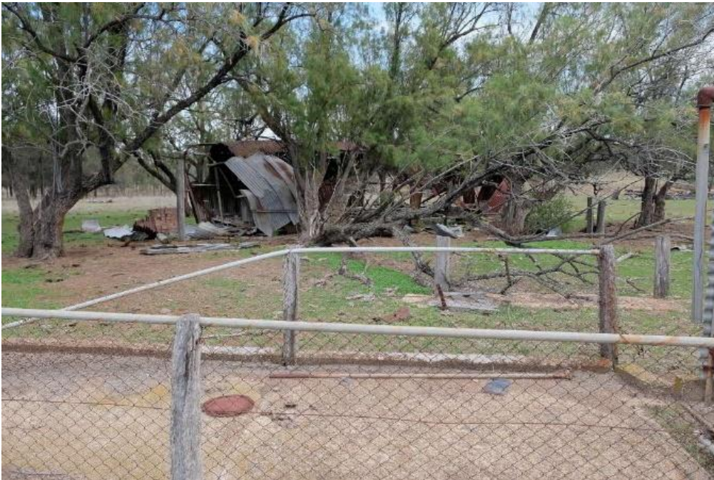
Figure 33 – View of concrete sheep run and yard in context with Nissen Hut.
