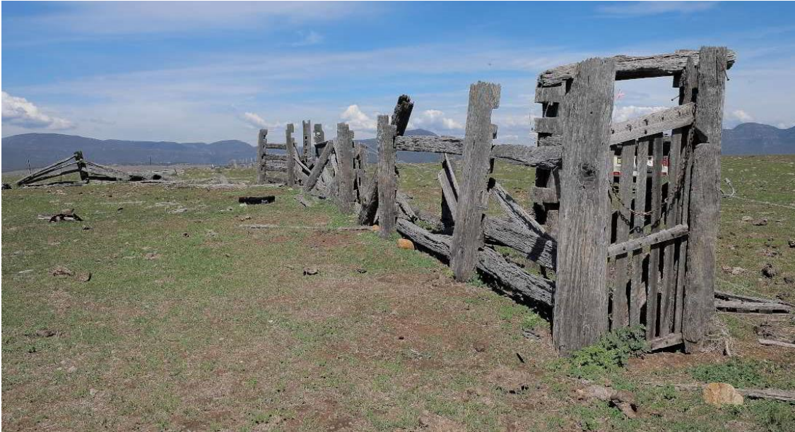
Figure 44 – View of the east-west run with the head beam connecting the two mid-posts.
