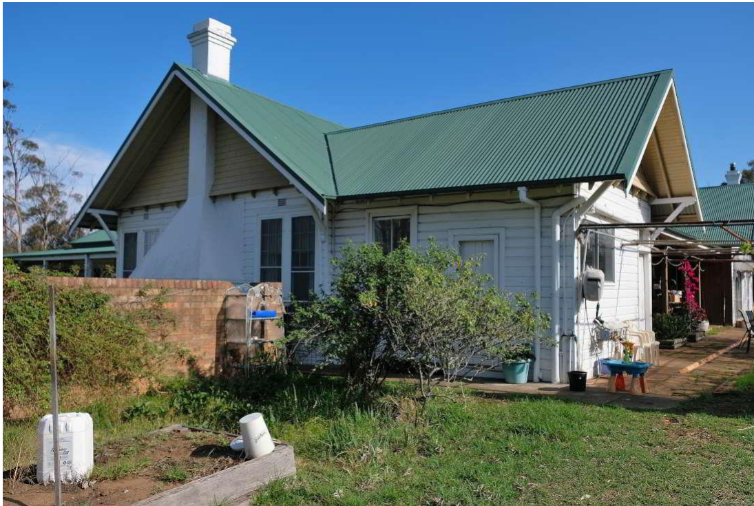
Figure 20 – View of north elevation showing the projecting gable with large rendered masonry fireplace.
