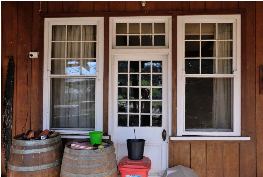
Figure 19 – View of east elevation under veranda, showing vertical clear finished timber cladding and white painted, multi-paned joinery.
