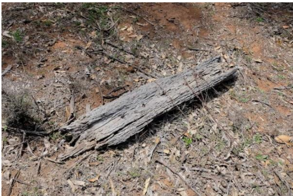
Figure 6 – Example of a fence post from M01 that differs from the typical timber post. Note it has no mortices for timber rails, only holes for wires, and is therefore likely to be a later replacement post.
