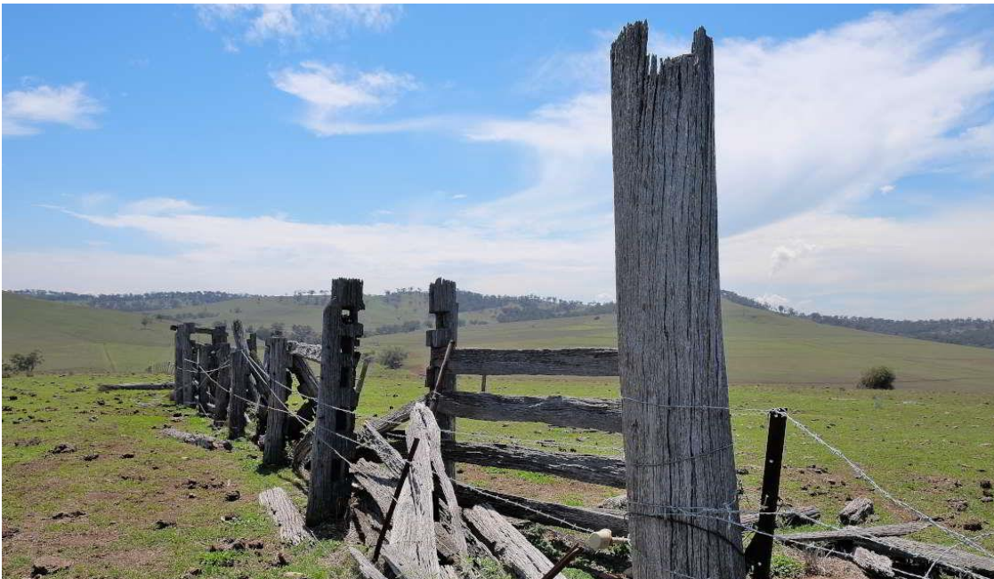
Figure 45 – View of the north-south run, looking from the southern end.
