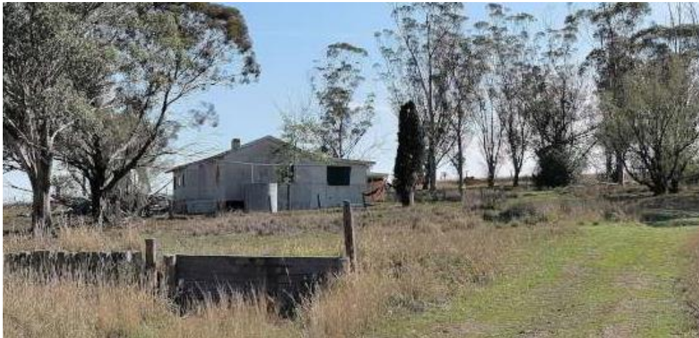
Figure 13 – One the timber houses located at some distance south-east of Edderton Homestead.
