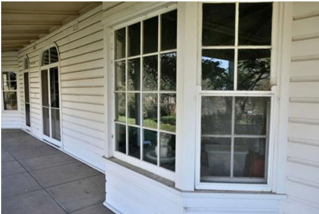
Figure 17 – Original front entry of Edderton Homestead. Note the doors have been modified with arched transom lights in a style similar to the interior detailing of the 1930s adaptations.
