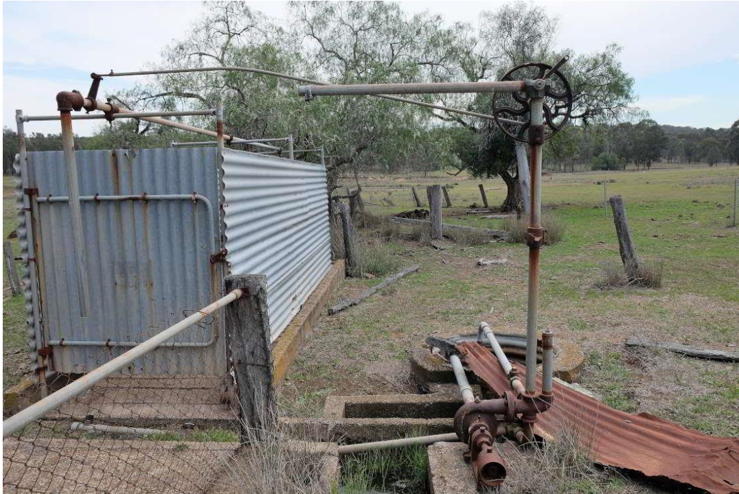
Figure 39 – The Cooper Type Sheep Shower elements surviving adjacent to the Nissen Hut. A concrete water tank and concrete-lined drainage channels sit adjacent to the enclosed showering area.
