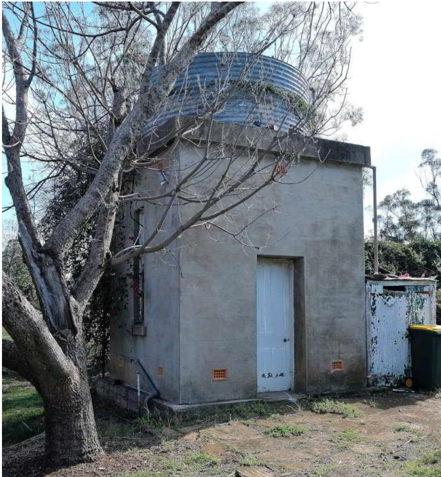
Figure 11 – The former dairy at Edderton constructed unusually in rendered masonry with a water tank.
