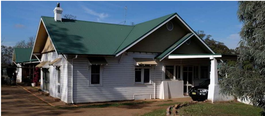
Figure 18 – View of south-east corner of Edderton Homestead showing the 'Porte Cochere' to the right and rear elevation to the left.
