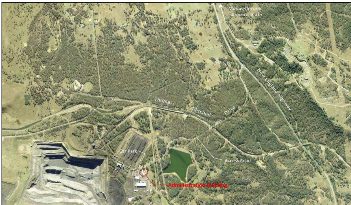
Figure 1: Location of Maxwell Administration Building
