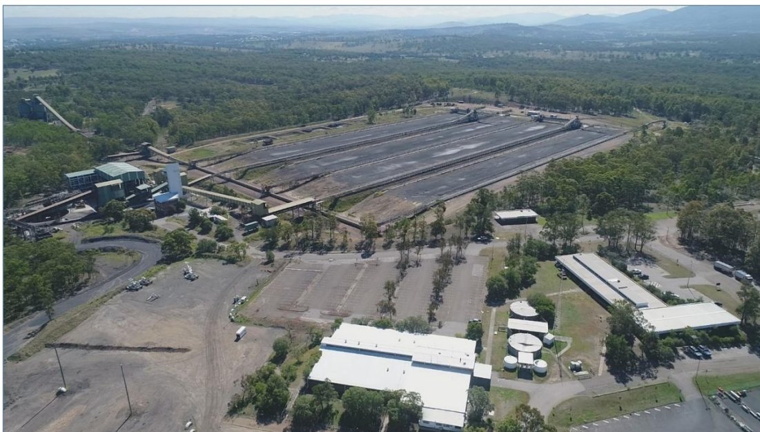
Plate 1-1 – Existing Maxwell Infrastructure
