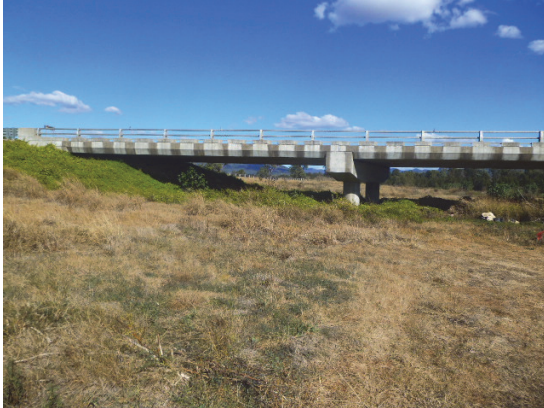
Fig. 6.4 Bridge across the floodplain adjacent to the Hunter River
