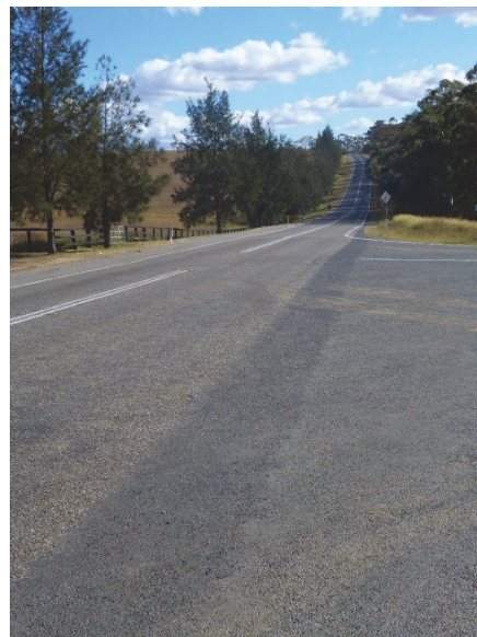
Fig. 6.1 The Golden Highway at the intersection with Edderton Road
