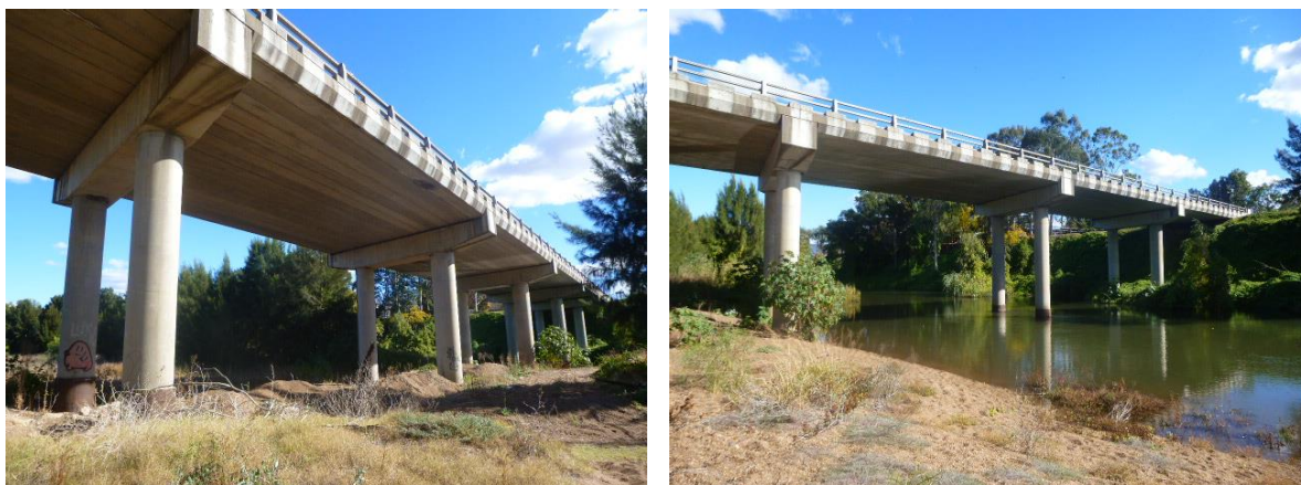
Fig. 6.3 Bridge where the Golden Highway crosses the Hunter River
