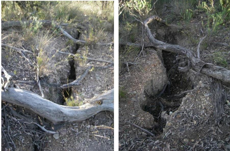
Fig. 4.6 Examples of surface cracking on steep slopes in the Hunter Coalfield
