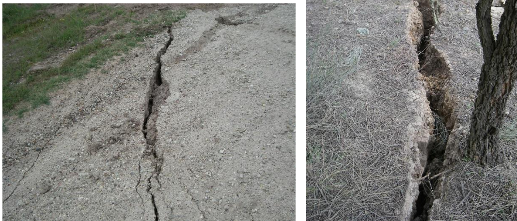
Fig. 4.5 Surface cracking above Blakefield South Mine (multi-seam conditions)
