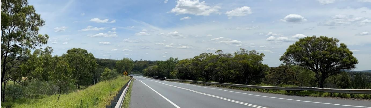
Figure 27. Current view from New England Highway
