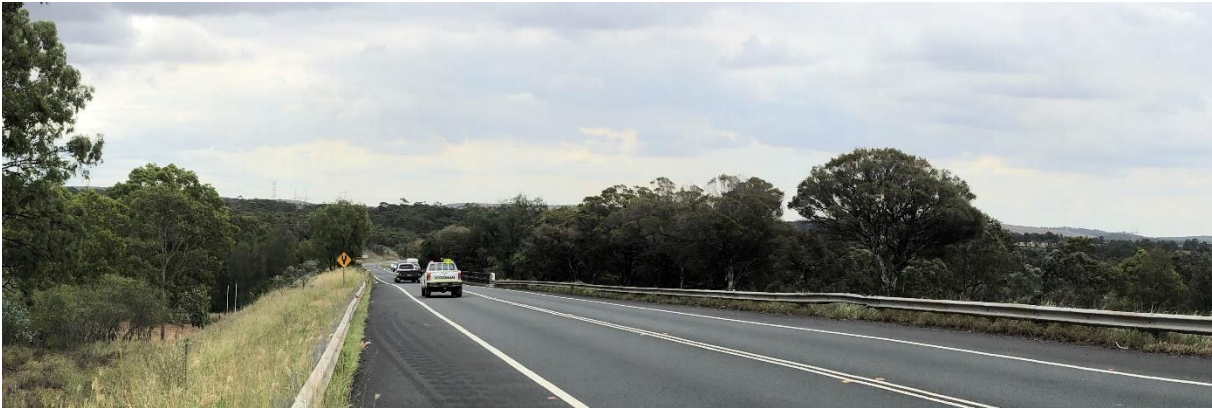
Figure 29. Current view from New England Highway
