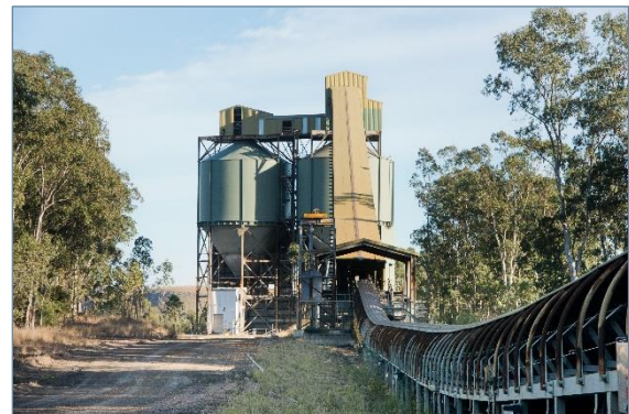
Plate 3-3 – Existing Train Load-out Facility
