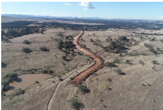
Plate 1: Construction of Initial Access Road
