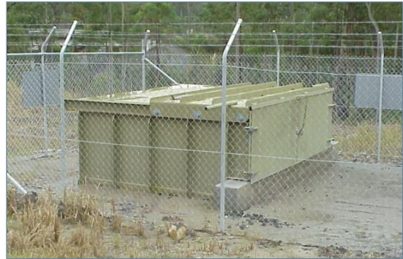
Plate 3-4 – Typical Service Borehole Site
