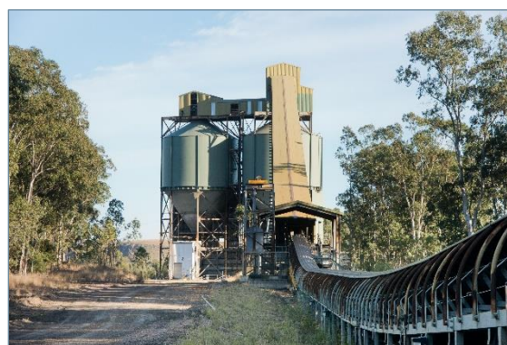
Plate 3-3 – Existing Train Load-out Facility
