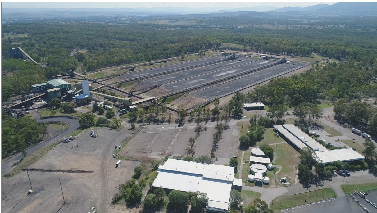
Plate ES-6 – Existing Maxwell Infrastructure
